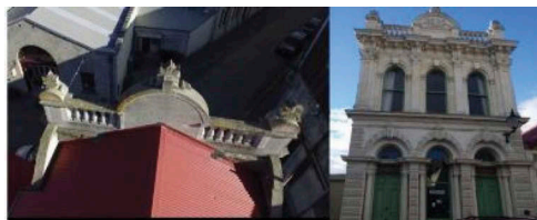
(g) Verification of no parapet restraints (Oamaru)
