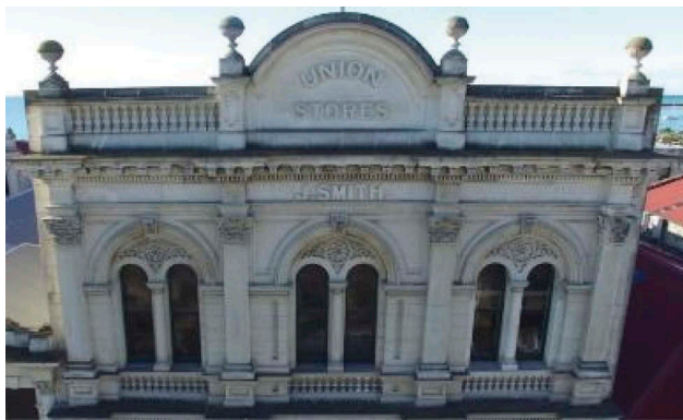
(a) Union Building, 7 Tyne Street, Oamaru
