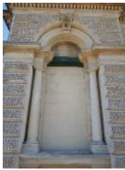
(a) Sealed openings (Oamaru)
