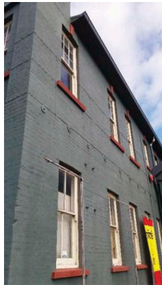
(a) Steel/wrought iron wall ties
