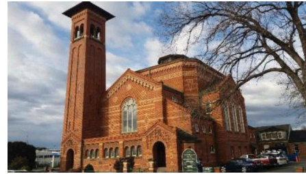
(e) Italo-Byzantine brick masonry
